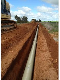
Flowtite GRP Pipe was chosen for this project due to a combination of high pressure capacity, high production rates, ease of installation and the chemical resistance of GRP.
