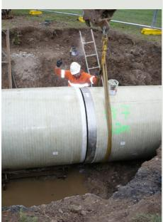
steel stormwater pipelines that had corroded and failed. The pipe route involved going under parklands with minimal cover height. Flowtite<sup>®</sup> Continuous Wound GRP Jacking Pipe was selected because it is light weight, could be customised to maximise internal diameter and does not corrode. Further, RPC Pipe Systems was able to nest the two diameters to minimise the cost of transportation.
